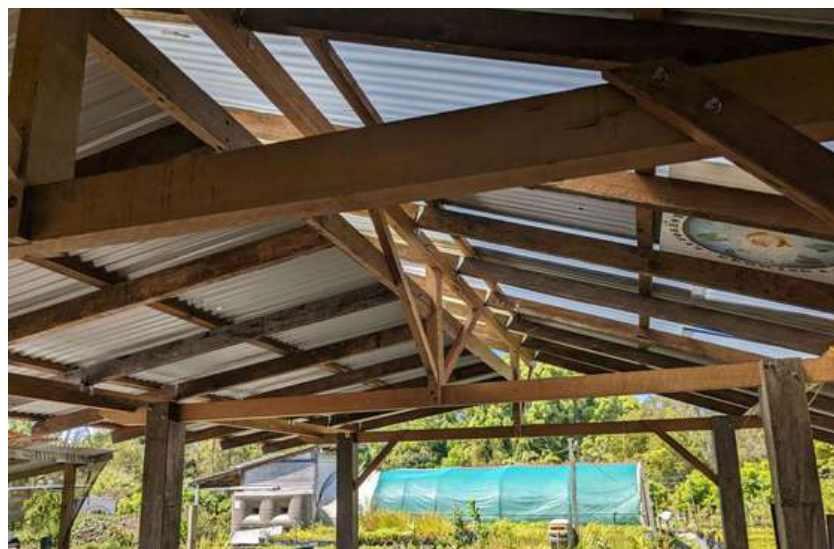
Clerestory roof design enables the light to pass through the middle of the workshop without allowing water to get in - a natural skylight.
